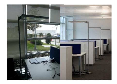
Figure 4.6.: Motion and daylight sensored lighting fixtures (February 2014)
