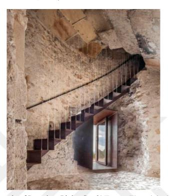
**Figure 2.3.** Example of Insertion: Pi des Catalá Tower. The original stone staircase and doorway has been replaced with a steel structure. Retrived from https://www.designboom.com/architecture/maria-castello-martinez-pi-des-catala-tower-restoration-formentera-spain
