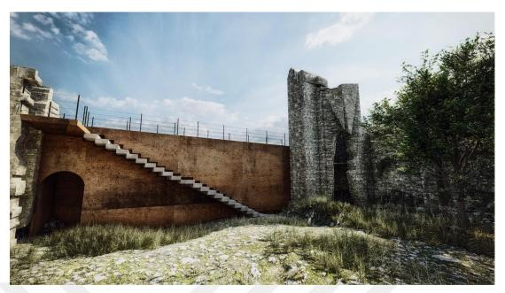
**Figure 4.8.** The view of the steel box extension and the concrete staircase from inside the castle interior.
