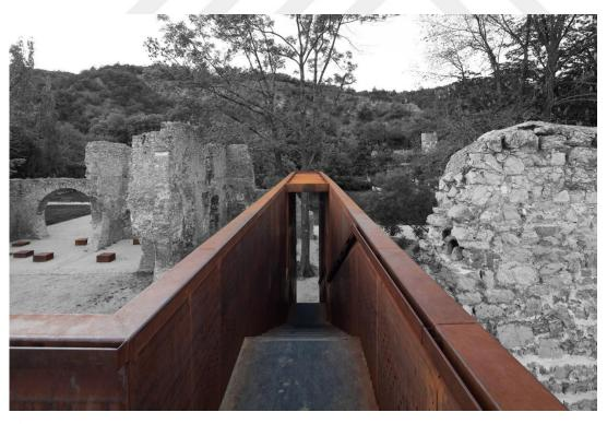
**Figure 3.7.** The circulation area of the contemporary addition applied with reference to the disappearing wall of the building. Retrieved from https://www.archdaily.com/272346/szatmary-palace-marp in October, 2021 and edited by the author.
