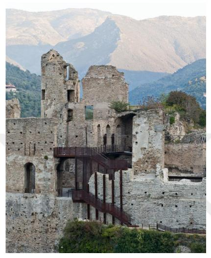
**Figure 3.32.** Contemporary staircase extension located in the place of the destroyed wall of the castle. Retrieved from https://www.archdaily.com/934655/restoration-of-castello-dei-doria-a-dolceacqua-ld-plus-sr-architetti in December, 2021
