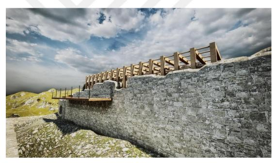
**Figure 4.13.** The steel balcony extension on the north wall of the inner castle and the pergola legs placed on the wall.
