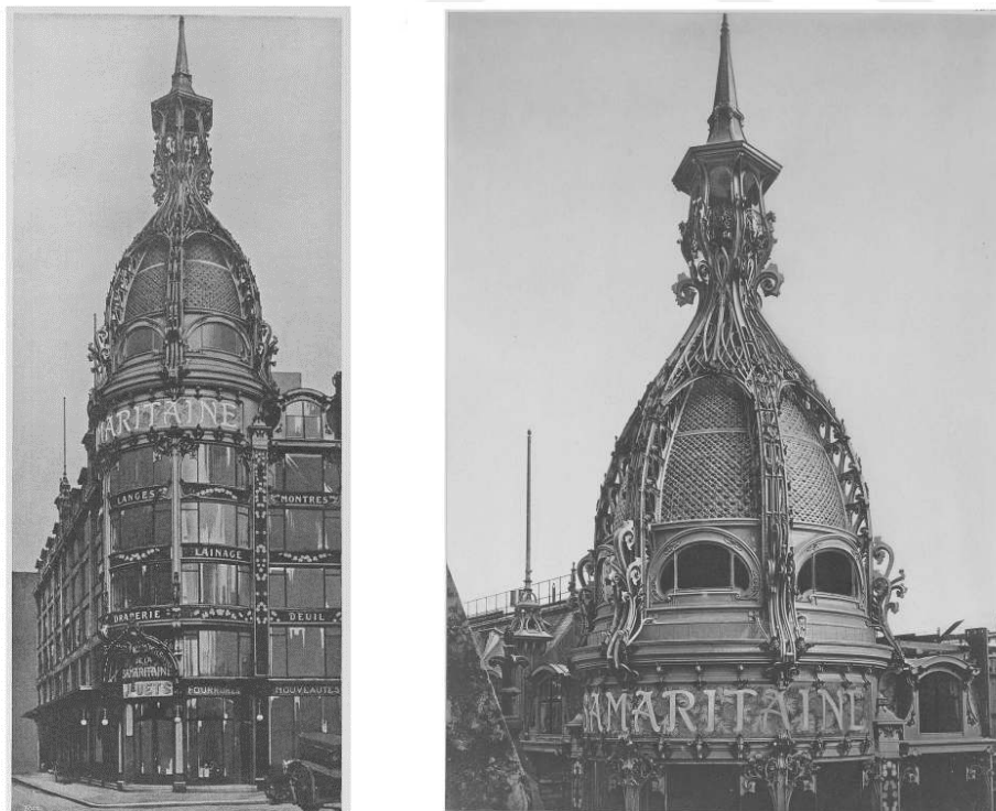
Figure 3.6. The Samaritaine renovated exterior (Vayron, 2015, p.6;13)
