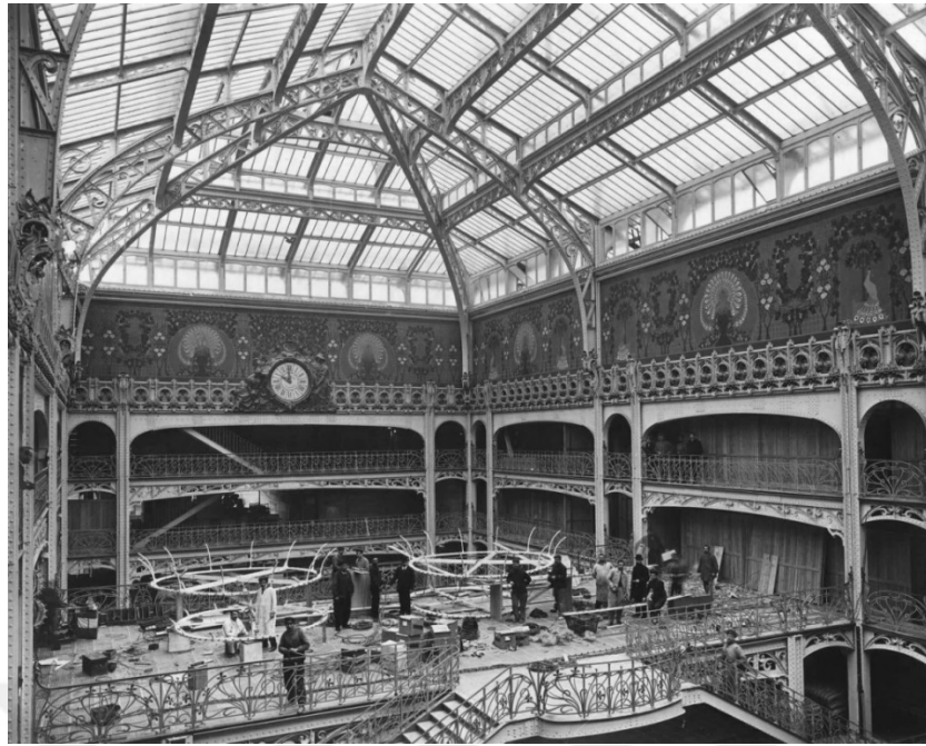
Figure 3.7. The interior of Samaritaine (Cabestan & Lempereur, 2011)
