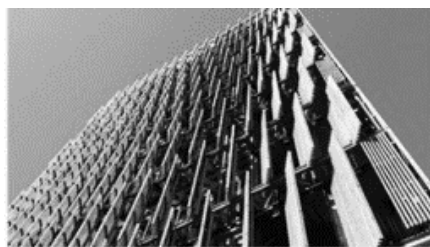
Council House 2 Building
