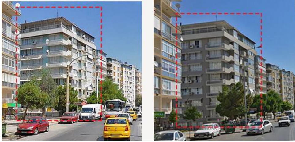
Figure 4.6. Kuğu Apartment with BTB façade, 2011; Kuğu Apartment after the sheathing work, 2015 (Yandex Map image, marked by the author)
