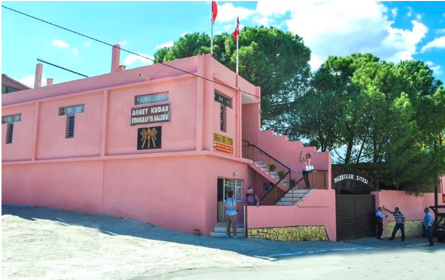
Figure 3.2 TAKEG building and the gallery garden in 2016 (Kaya, 2016)
