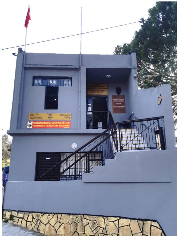
Figure 4.33 The front facade of TAKEG (Author's Photo Archive, 2018)
