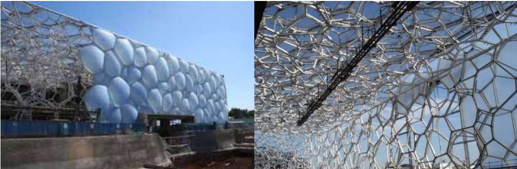
Figure 3.12. Water cube, Beijing
