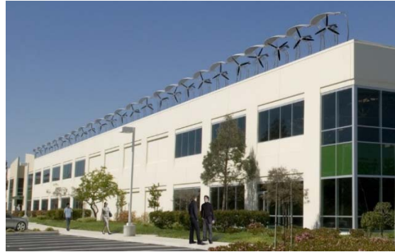
Figure 3.27. Integration of micro-wind turbines into urban area as a built environment (Climate Technology Centre and Network, n.d.)
