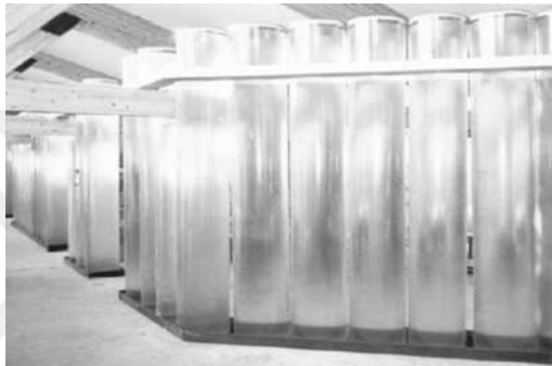
Figure 3 Solar Components Water Wall (Bainbridge, 1981)
