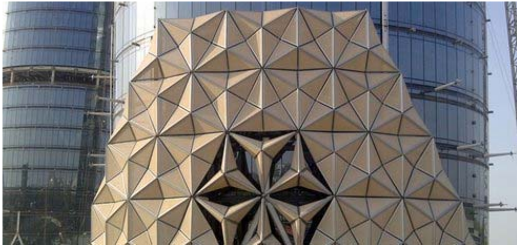
Figure 13 Al-Bahar Tower Responsive Kinetic Shading Devices (“Al-Bahar Tower Facade,” n.d.)
