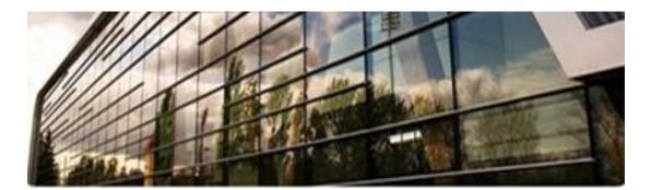
*Figure 16: Curtain Wall System* Source: (Al Dakheel, J. and Tabet Aoul, 2017)
