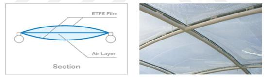
*Figure 31: Triple layered ETFE* Source: (Sert, 2016)
