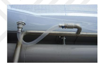
Figure 27: ETFE Cushion Air Valve Source:(Moritz, 2007)
