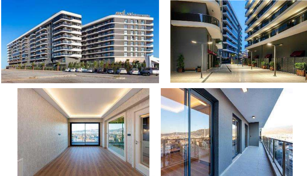
Figure 4.8. Exterior and interior views of the project (Source: Caddebostan, 2021)
