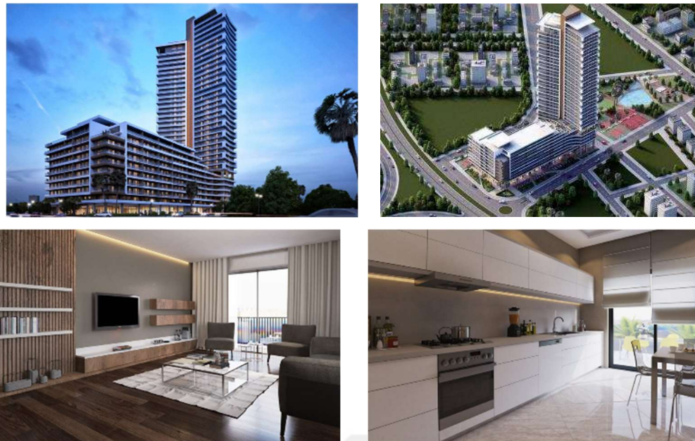
Figure 4.59. Exterior and interior views of the project (Source: İkon Tower, 2021)
