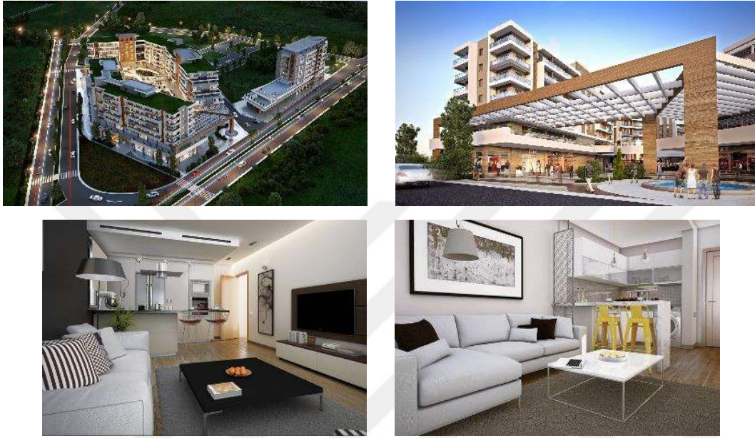
Figure 4.83. Exterior and interior views of the project (Source: MyVia 414, 2021)
