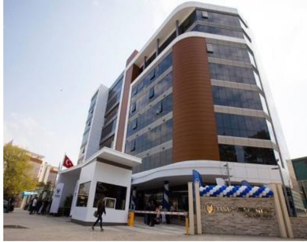
Figure 3.5. The T building has four façades (Image: Yildirim, Gundogdu, & Kahraman, 2019).
