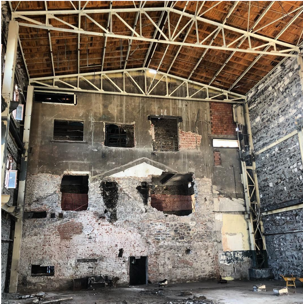
Figure 88 Interior of the Yaşar Museum before the intervention, Alsancak, İzmir.
