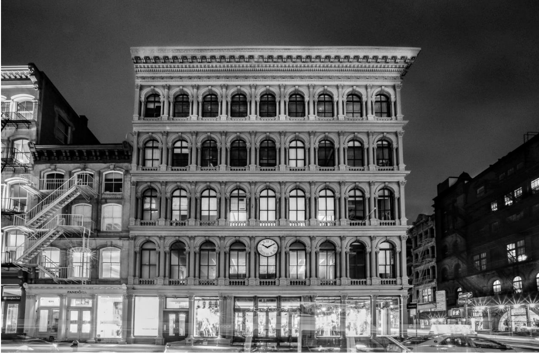
Figure 16 488 Broadway, Manhattan E. V. Haughwout Building
