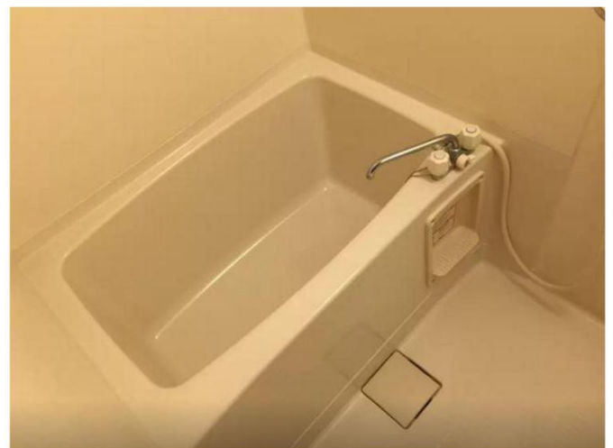
Figure 2.28 Site Pictures of the sink, toilet and bathing areas (Takumi Japan, 2014)
