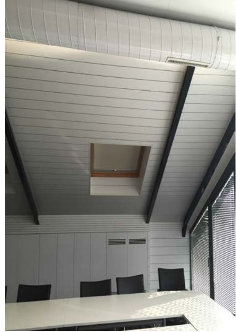
Figure 4.34: the Roof Windows (Idil BAKIR Photo Archive,2015)
