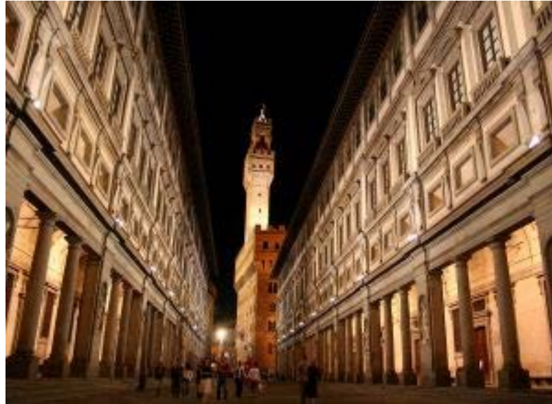
Figure 2.1 : Uffizi Palace External View
