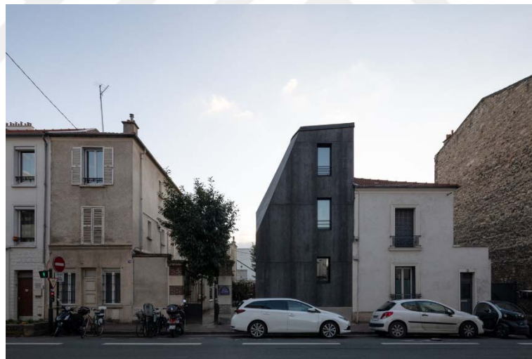
Figure 4.6 Example of Continuity. Retrieved from: https://www.archdaily.com/932524/house-v-tectone?ad_source=search&ad_medium=projects_tab in December, 2021
