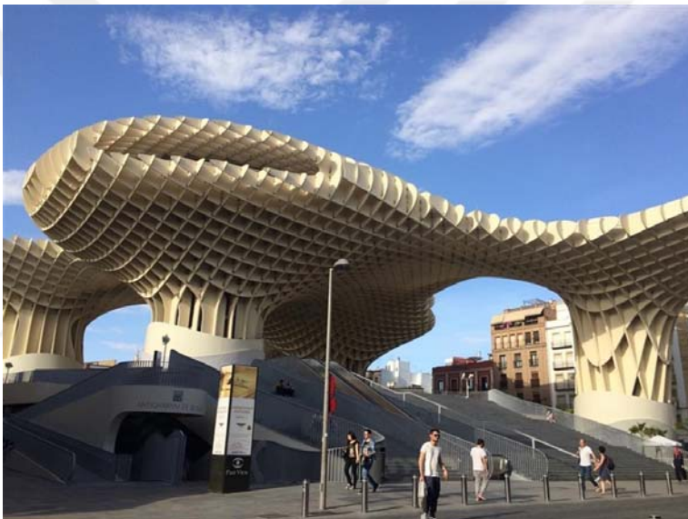
Figure 4.10 Evaluation of Simplicity in Form, Metropol Parasol. Retrieved from: https://www.archdaily.com/201961/metropol-parasol-j-mayer-h-arup in December, 2021
