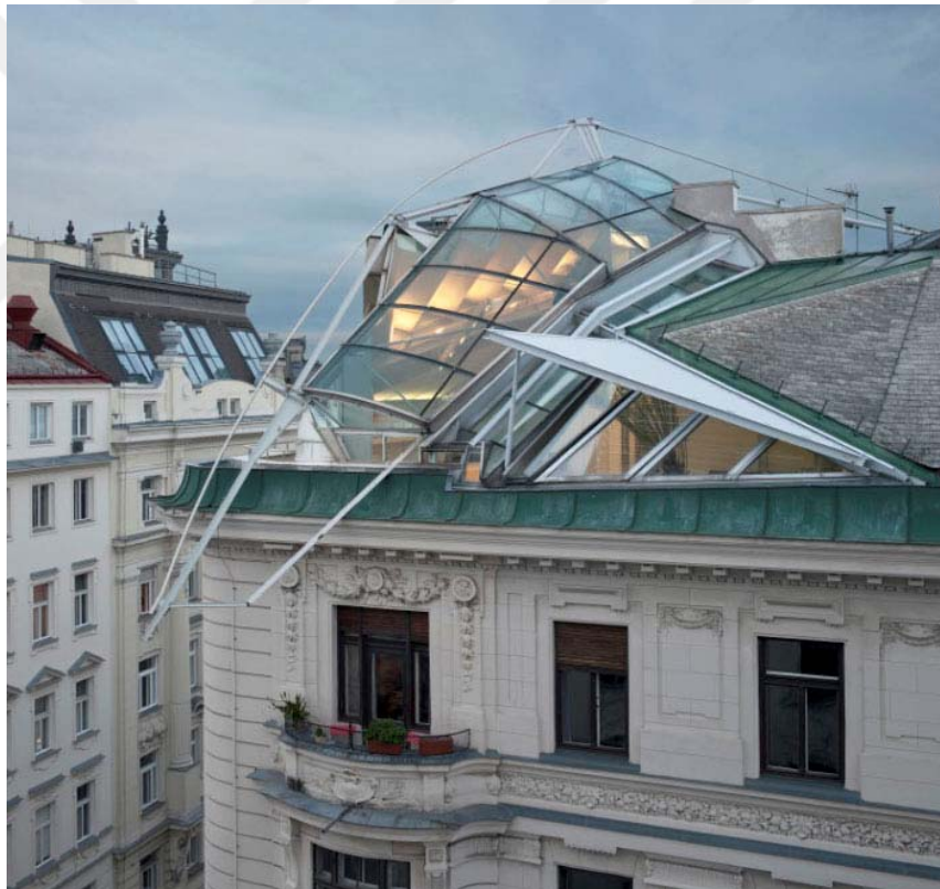
Figure 5.4 A view from Falkenstrasse 6 Addition. Retrieved from: http://www.coop-himmelblau.at/architecture/projects/rooftop-remodeling-falkestrasse/ in December, 2021
