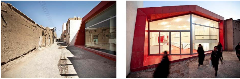
Figure 4.16 Views of No name Shope. Retrieved from: https://www.archdaily.com/287306/no-name-shop-iranian-architectural-atelier in March, 2020.
