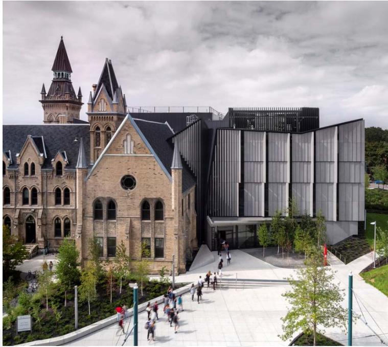
Fig. 4.7 Daniel Buildings and historical Building. Retrieved from: https://www.archdaily.com/916301/daniels-building-at-university-of-toronto-nadaaa in March, 2019.
