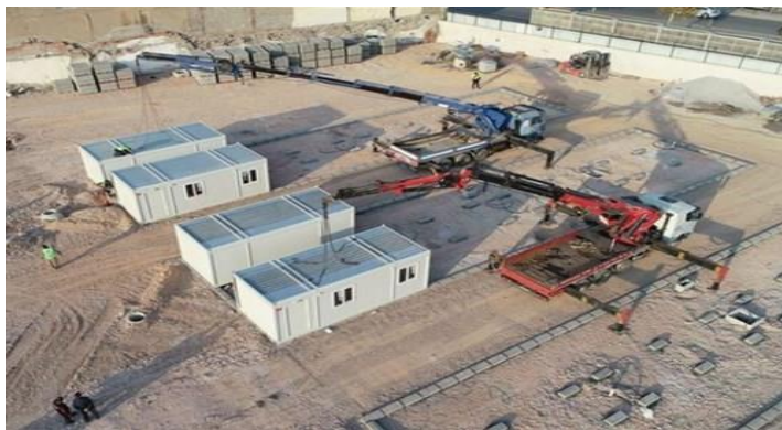
Figure 3.5. Container Housing Camp
