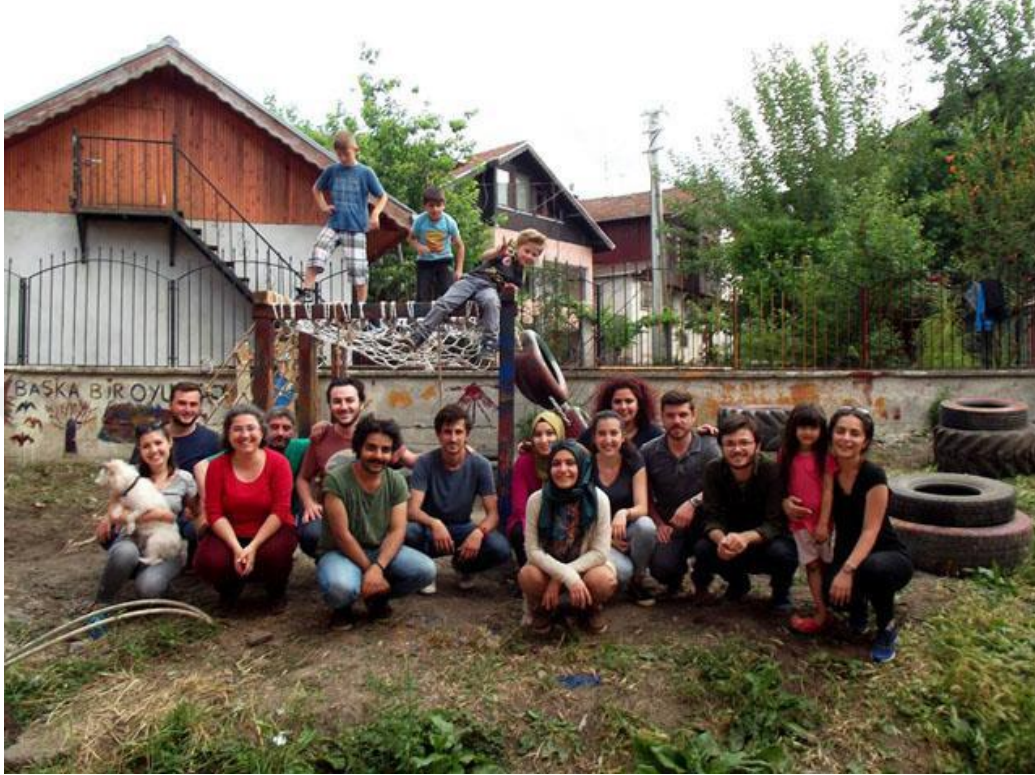
Figure 7. Başka Bir Atölye and the children of Saraylı village, an experimental playground design and construction by waste materials with the participation of users, Başka Bir Oyun, Kocaeli, 2016.
