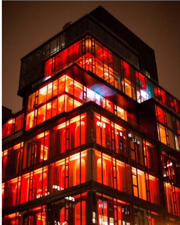
Figure 4.47. 15 West Union Square at Night Retrieved From: https://www.walksofnewyork.com/blog/urban-renewal-old-tiffany-gets-a-makeover
