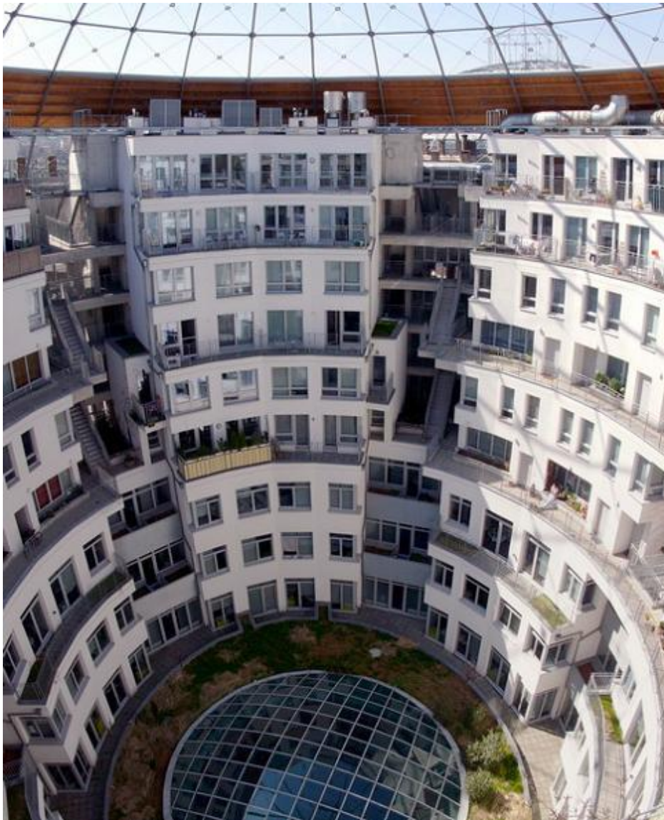
Figure 4.87. Interior of the Gasometers Retrieved from: https://twistedstifer.com/2009/10/gasometers-of-vienna/
