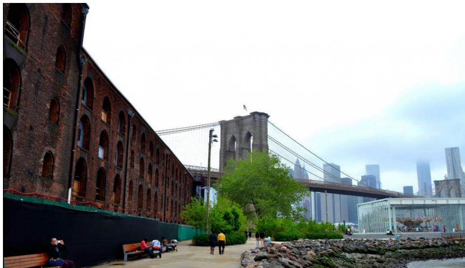
Figure 4.33. Waterfront Side of Empire Stores in 2014 During Construction
