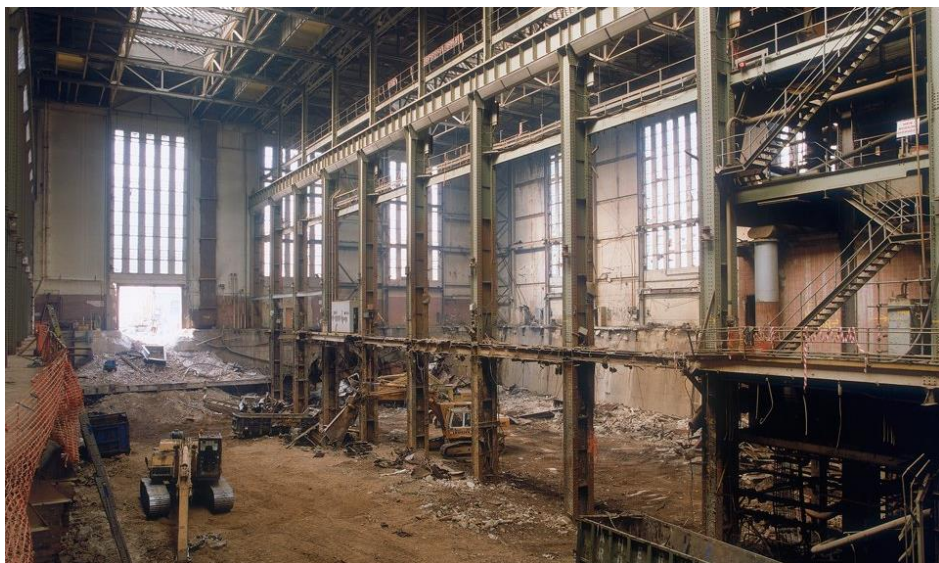
Figure 4.75. Demolition of the interior of the turbine hall Retrieved from: https://www.tate.org.uk/visit/tate-modern/look-behind-art-tate-modern
