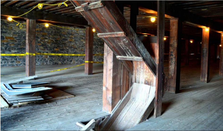
Figure 4.37. Wooden Chute for Sliding Coffee bean Bags Retrieved from: https://brooklyneagle.com/articles/2014/05/21/empire-state-of-mind-inside-the-iconic-empire-stores-warehouses/
