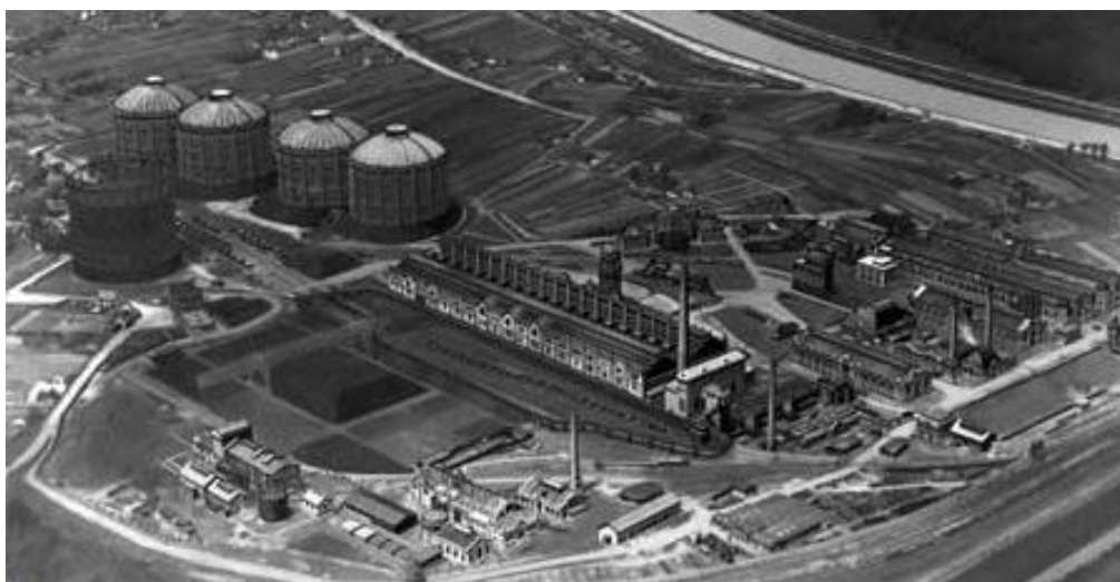
Figure 4.85. Simmering District aerial Retrieved from: https://www.atlasobscura.com/places/gasometer-town
