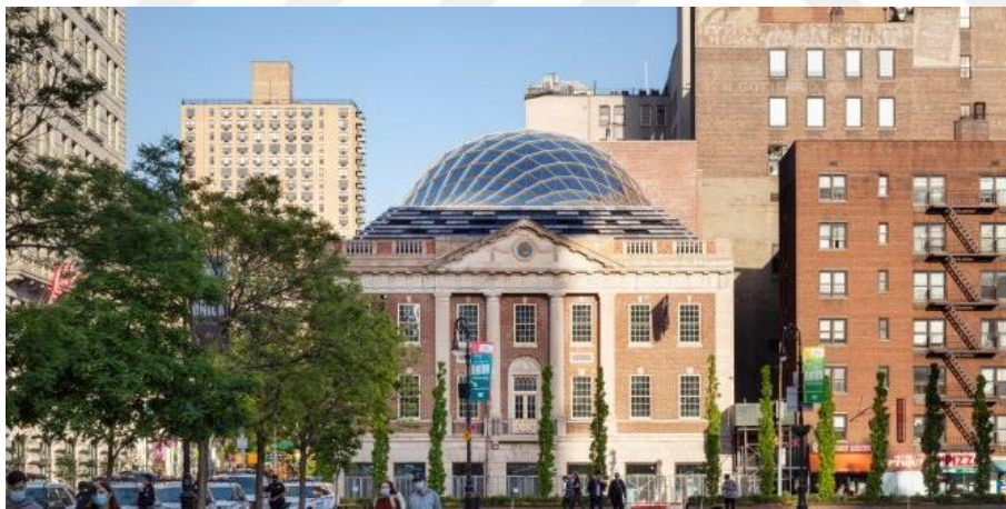
Figure 4.11. Street View of the Building after Renovation Retrieved from:
