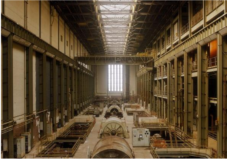
Figure 4.74. The initial turbine hall Retrieved from: https://www.tate.org.uk/visit/tate-modern/look-behind-art-tate-modern
