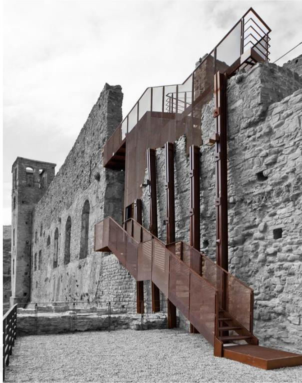
**Figure 3.36.** Metal staircase addition that allows circulation between the different levels of the castle. Retrieved from <https://www.archdaily.com/934655/restoration-of-castello-dei-doria-a-dolceacqua-ld-plus-sr-architetti> in December, 2021 and edited by the author.
