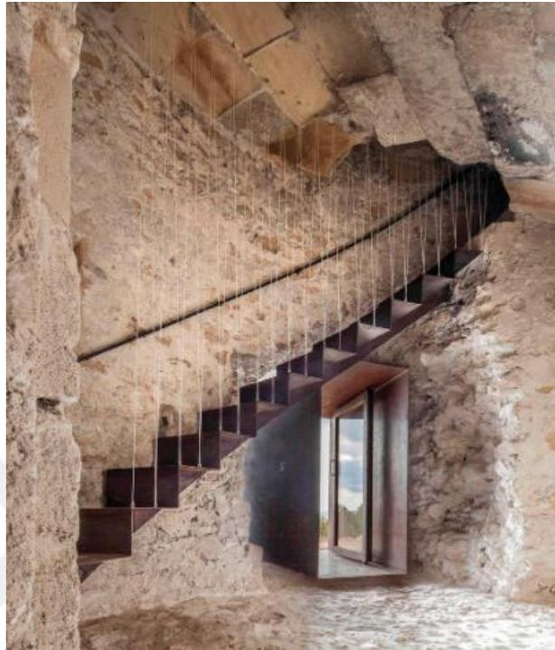
**Figure 2.3.** Example of Insertion: Pi des Catalá Tower. The original stone staircase and doorway has been replaced with a steel structure. Retrieved from <https://www.designboom.com/architecture/maria-castello-martinez-pi-des-catala-tower-restoration-formentera-spain>
