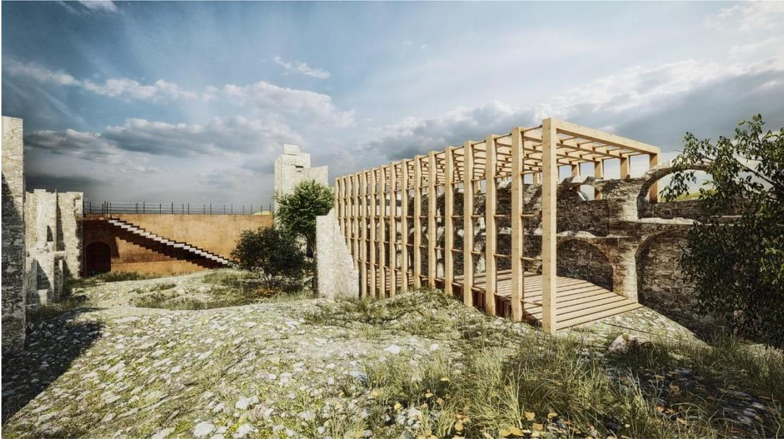
**Figure 4.10.** Addition of pergola and wooden flooring defining the ward area and steel box addition at the back.
