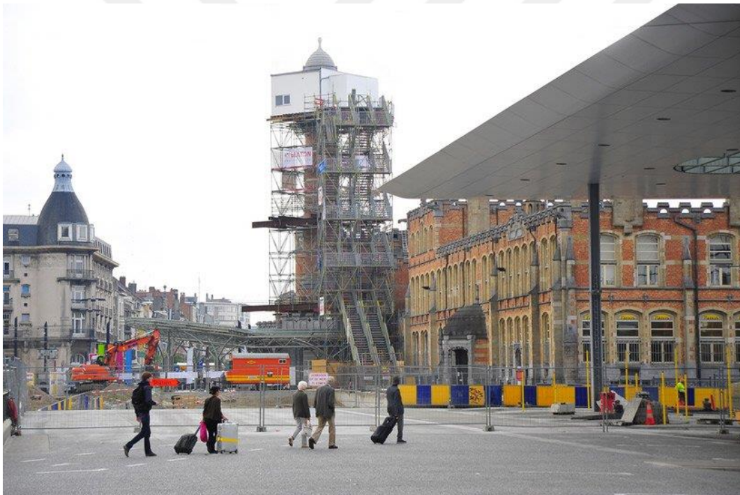
Figure 3.47. New silhouette of train station and clock tower with Hotel Gent project. Retrieved from https://www.designboom.com/art/tazu-rous-aka-tatzu-nishi-temporary-belltower-hotel-in-ghent/ in December, 2020
