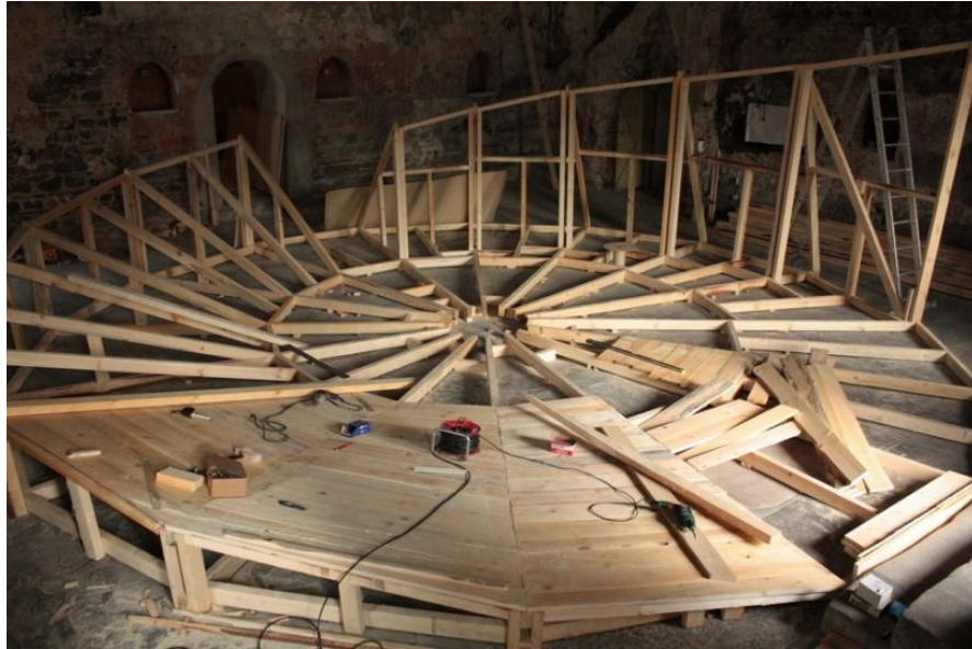
Figure 3.20. Structure of |CON|Temporary Library. Retrieved from: https://studio812.eu/portfolio/con-temporary-library/ in March, 2020.
