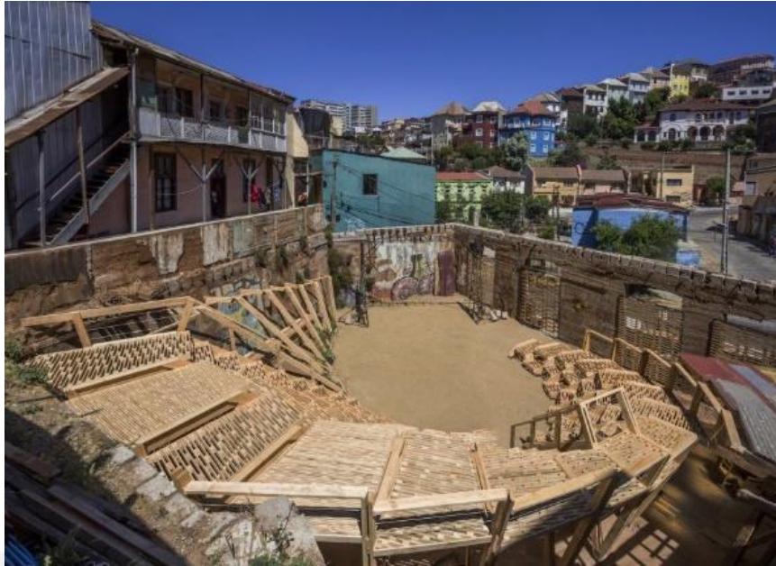
Figure 3.48. New amphitheater structure of The Wave project. https://inhabitat.com/the-wave-an-abandoned-urban-lot-is-revived-as-a-thriving-performance-arts-space/ in December, 2020
