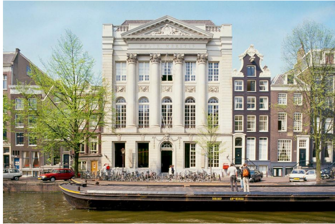
Figure 3.26. Felix Meritis Building exterior view. Retrieved from: http://ttnotes.com/felix-meritis-cultural-center.html in September, 2020.
