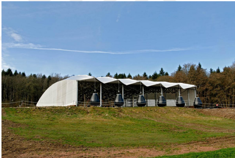
Figure 3.53. Filled black canvas bags for rain resistance system. Retrieved from https://www.tess.fr/en/projet/excavation-shelter# in December, 2020
