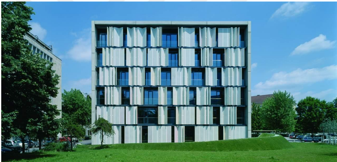
Figure 2.12. Biocatalysis Lab Building at Technical University Graz (Ott, 2004)
