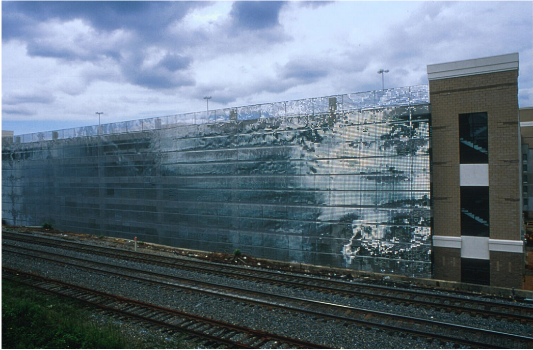
Figure 2.30. Charlotte Parking Garage (Kahn, 2019)
