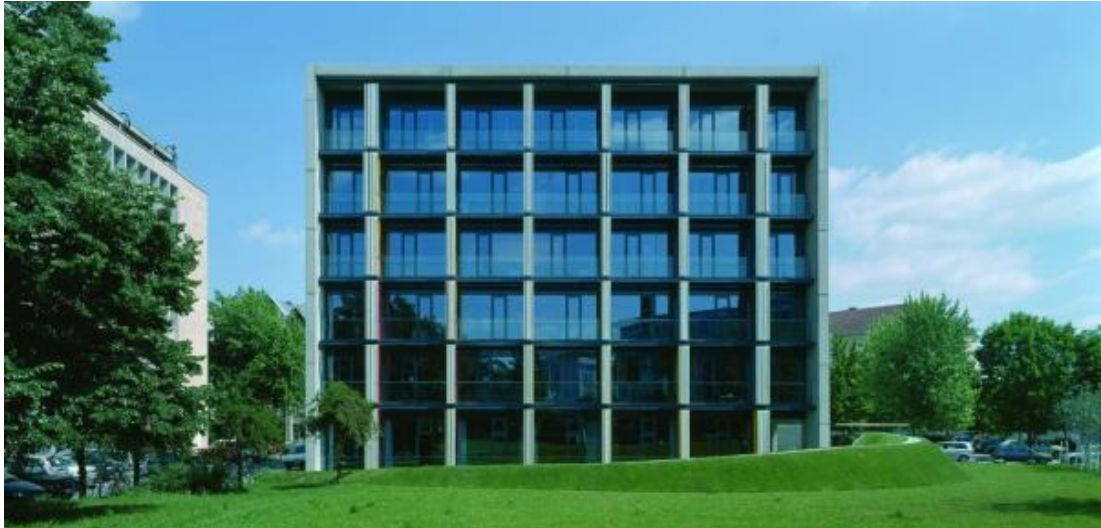
Figure 2.11. Biocatalysis Lab Building at Technical University Graz (Ott, 2004)
