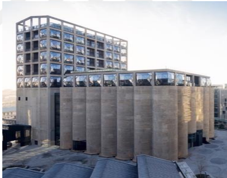
Figure 3.31: Contemporary structures' exterior façade after the intervention.
