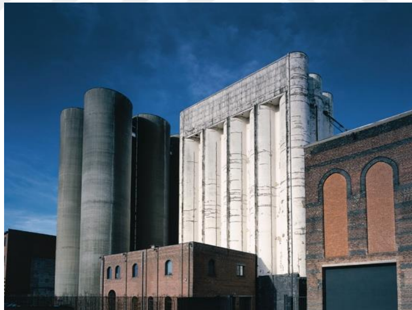
Figure 3.36: Authentic structure before intervention.
