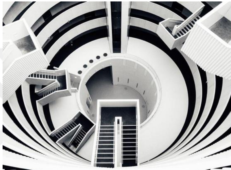
Figure 3.18: Circulation axis consisting of stairs, corridors and elevators formed inside the silo structures. Retrieved from https://photorator.com/photo/83302/inside-the-gemini-residence-converted-into-a-residential-building-from-two-silos-by-mvrdv-copenhagen- in 13.06.2019
