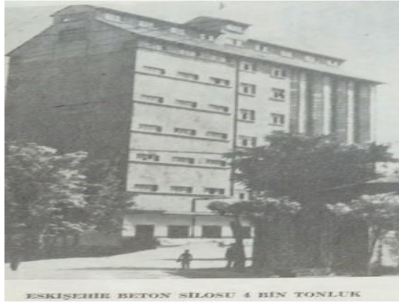
Figure 3.55: Picture showing the first years of the structure, obtained from the archive of TMO. Turkish Grain Board 1938-1959, 1959, Ankara: It was extracted from the work published by Turkish Grain Board. Copyright Owner is Turkish Grain Board.
