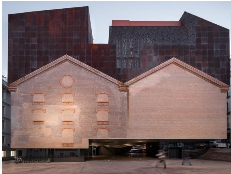
Figure 2.15: Re-functionalized contemporary building. Retrieved from: https://www.e-architect.co.uk/madrid/caixa-forum on 14.05.2019
