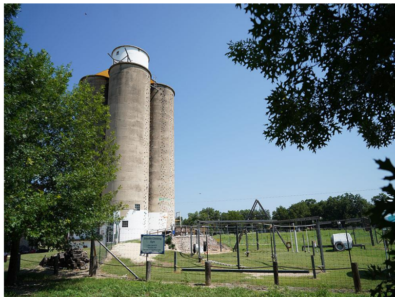
Figure 3.12: Newly formed exterior façade of the climbing silo after the intervention.
