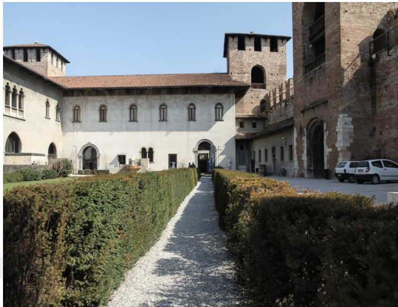
Figure 2.1: View from the central courtyard of Castelvecchio
