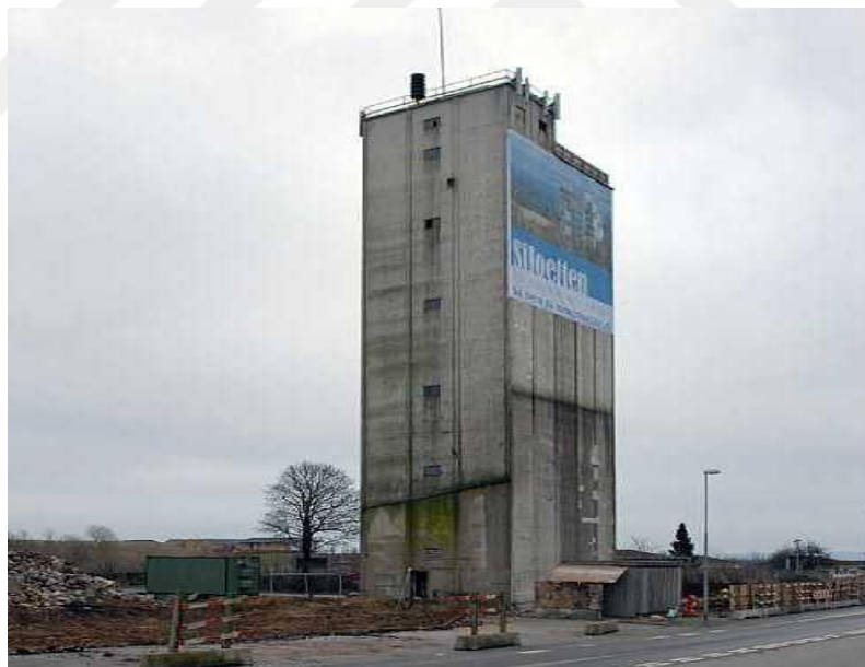
Figure 3.24: Authentic silo structure.
