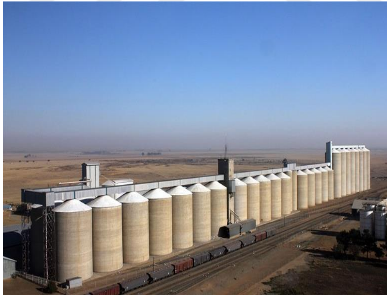
Figure 3.6: World's largest reinforced concrete silo with a capacity of 275.000 tons located in South Africa Retrieved from https://www.xtraspace.co.za/blog/articles/five-of-the-worlds-biggest-storage-spaces-no5 in 16.09.2019
