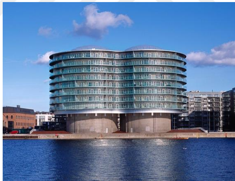
Figure 3.17: Contemporary living spaces created with intervention on the exterior façade of the authentic structures.
