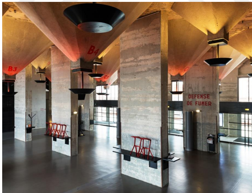
Figure 3.45: Art gallery where the funnels under the silos, which were completely emptied by the intervention, were created by preserving them. Retrieved from http://www.philippeconti.com/nav.php?root=data&proj_nb=1&photo_nb=0 in 27.11.2019.
