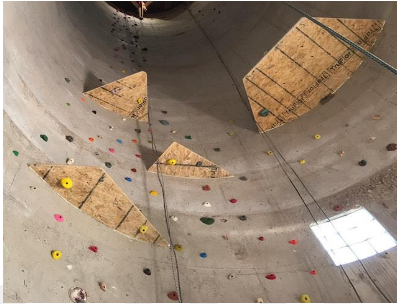
Figure 3.13: Newly attached climbing modules inside the climbing silo after the intervention.
