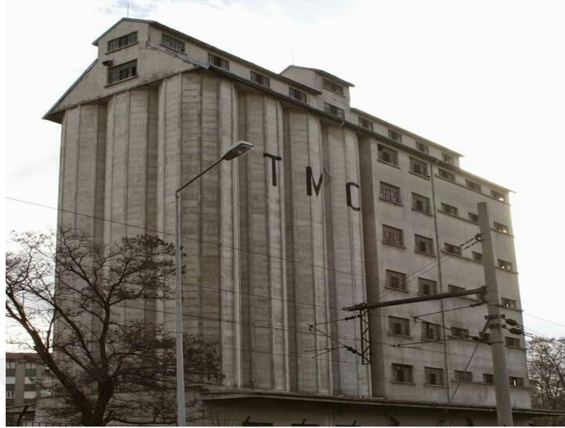
Figure 3.56: Authentic structure before the intervention.
