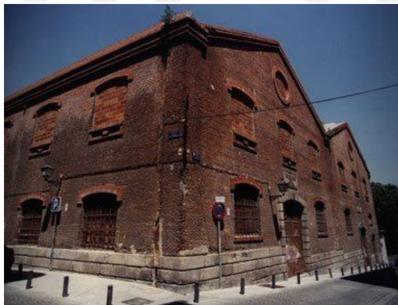
Figure 2.14: Authentic electric factory building.
