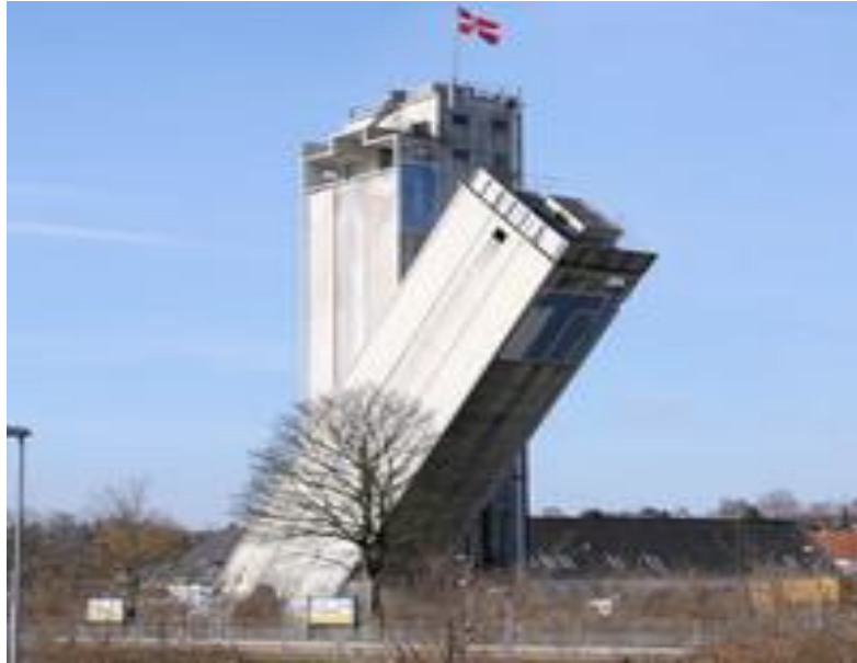
Figure 3.23: Demolition of one of the authentic silos.
