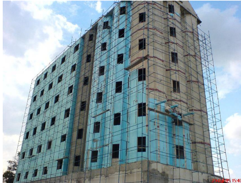
Figure 3.57: Heat insulation installation to the exterior façade during the intervention phase.
