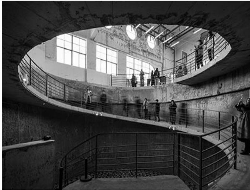
Figure 3.64: Spiral ramp built into one of the silos.
