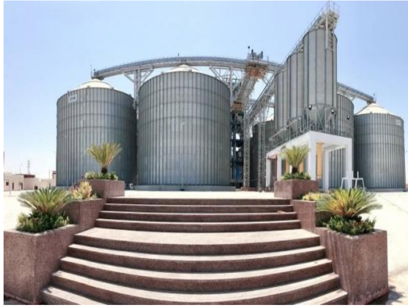
Figure 3.7: World's largest steel silo facility with a capacity of 1,3 million tons located in Egypt.
