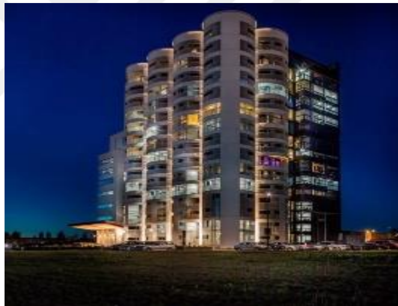
Figure 3.10: New construction after authentic structures were demolished. Retrieved from http://www.siilot.fi/kuvia/ in 24.05.2019
