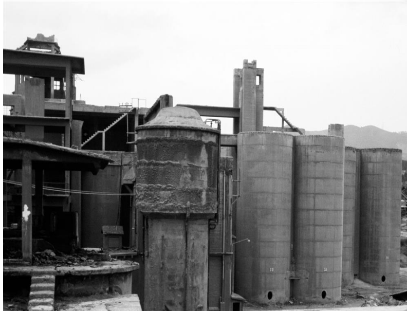
Figure 3.49: Authentic silo structure.
