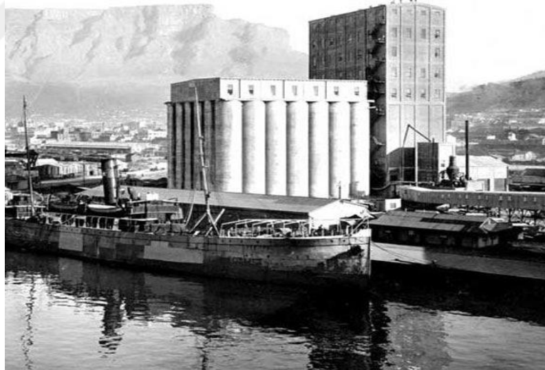
Figure 3.30: Authentic silo structure,
