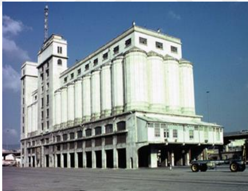
Figure 3.42: Authentic silo structure.
