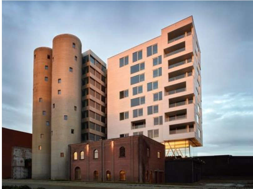
Figure 3.37: Contemporary structure after the intervention.
