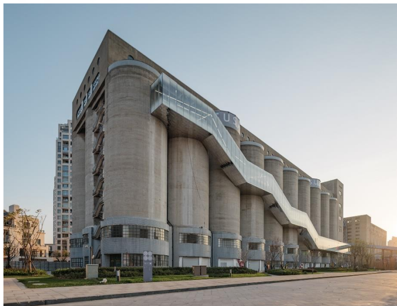
Figure 3.63: Circulation axis created by intervention to the outer shell of the contemporary structure.
