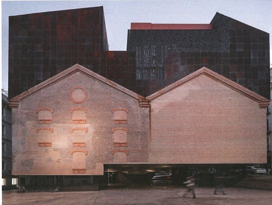
Figure 2.7. Herzog & de Meron's intervention on Caixa Forum (Lomholt, 2018).
