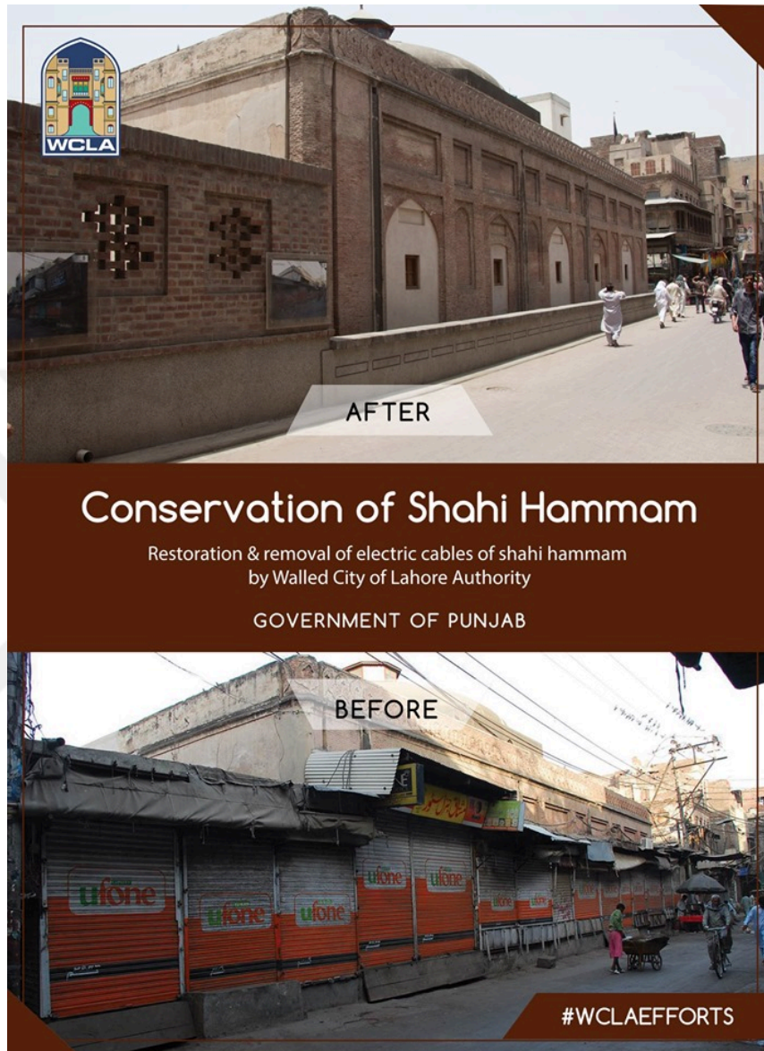
Fig 3.7: Restoration of Shahi Hammam (Before and After)
